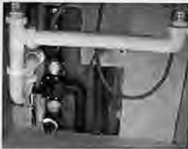
A three-way diverter valve is spliced in under a kitchen sink. Note that the incoming line from the kitchen sinks had to be raised to make space.
