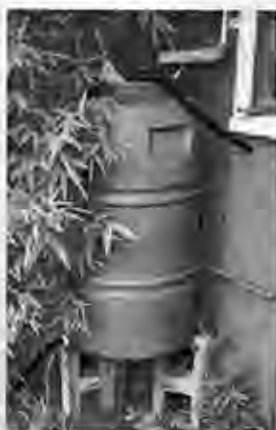
A "gravity drum" supplied by washer drain hose run through a 1" hole in the wall. Note this drum also catches rain water, which runs through a screen mesh and out through the same hose to flush salts from the mulch basins.
