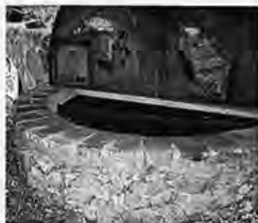
Beautifully made but ill-conceived greywater storage tank. This four foot wide, four foot deep tank is the final of a four-chamber system which converts greywater to foul-smelling blackwater over the course of the week it takes to get through the system. The water is dark black, smells vicious, and generates hydrogen sulfide which has eaten through the steel lid.
