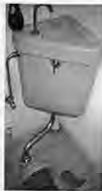
Water is used for washing hands before it flushes the toilet in a common Japanese fixture
